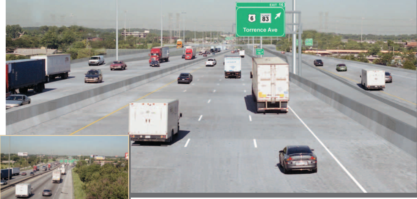
I-80/94 (Kingery Expressway) heading east on approach to Torrence Ave. (Ill. Rte. 83)
